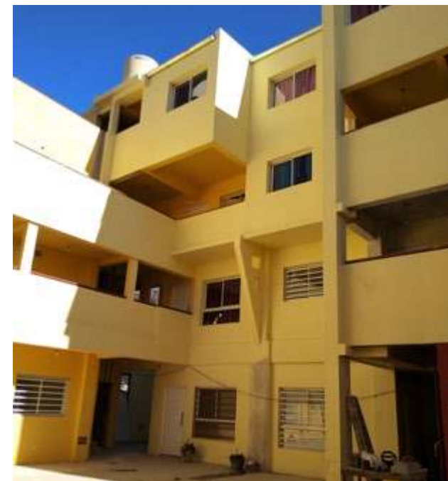
Patio central interno
